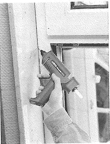
Sealing joints.
